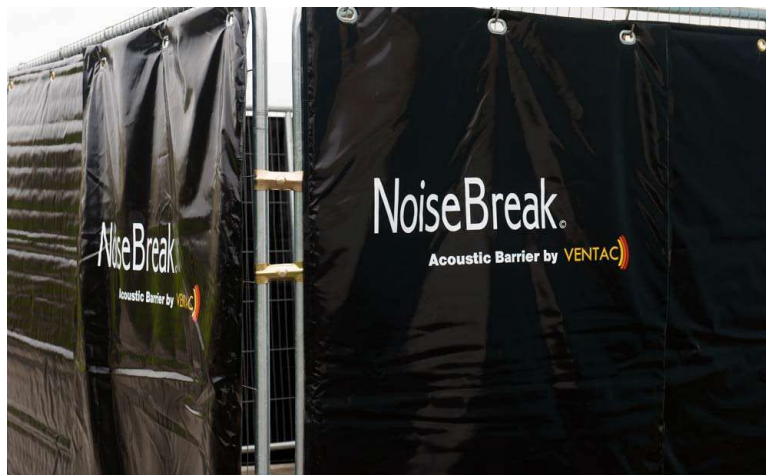
Figure 13.4: Temporary construction noise barrier © Ventac
